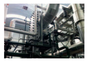
In the Miajadas plant, the main duty of these Compabloc units is to use extraction steam from the turbine to heat the boiler water from 50°C to 80–90°C. According to Rafael Godoy, "This equipment, which has been designed specifically to suit our needs, provides outstanding performance as well as being very compact." This space-saving design then made it possible to mount this pre-heater unit in the most convenient place.
