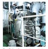
PureBallast 3 reactor integrated into pipework after installation.
