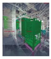
3D laser scans allowing exact positioning of PureBallast 3 components.
